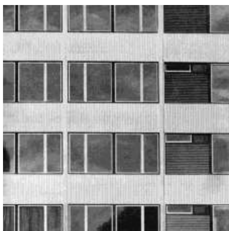
Figure 2: Front of Jugomont's residential building JU-61 (** 1962).
