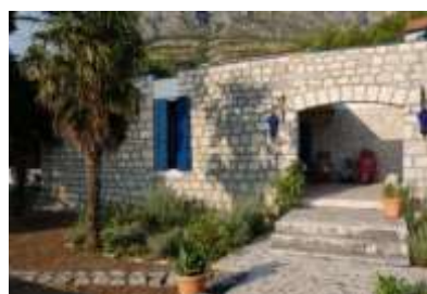
Figure 2: View from the west.
